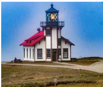
Lighthouse with ARC used
